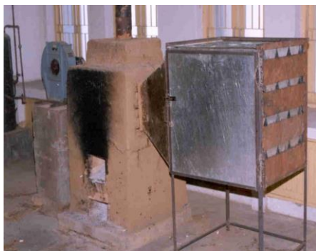
Waste fired dryer
